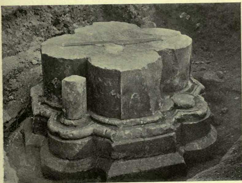
BASES OF PIERS, NAVE ARCADE.
