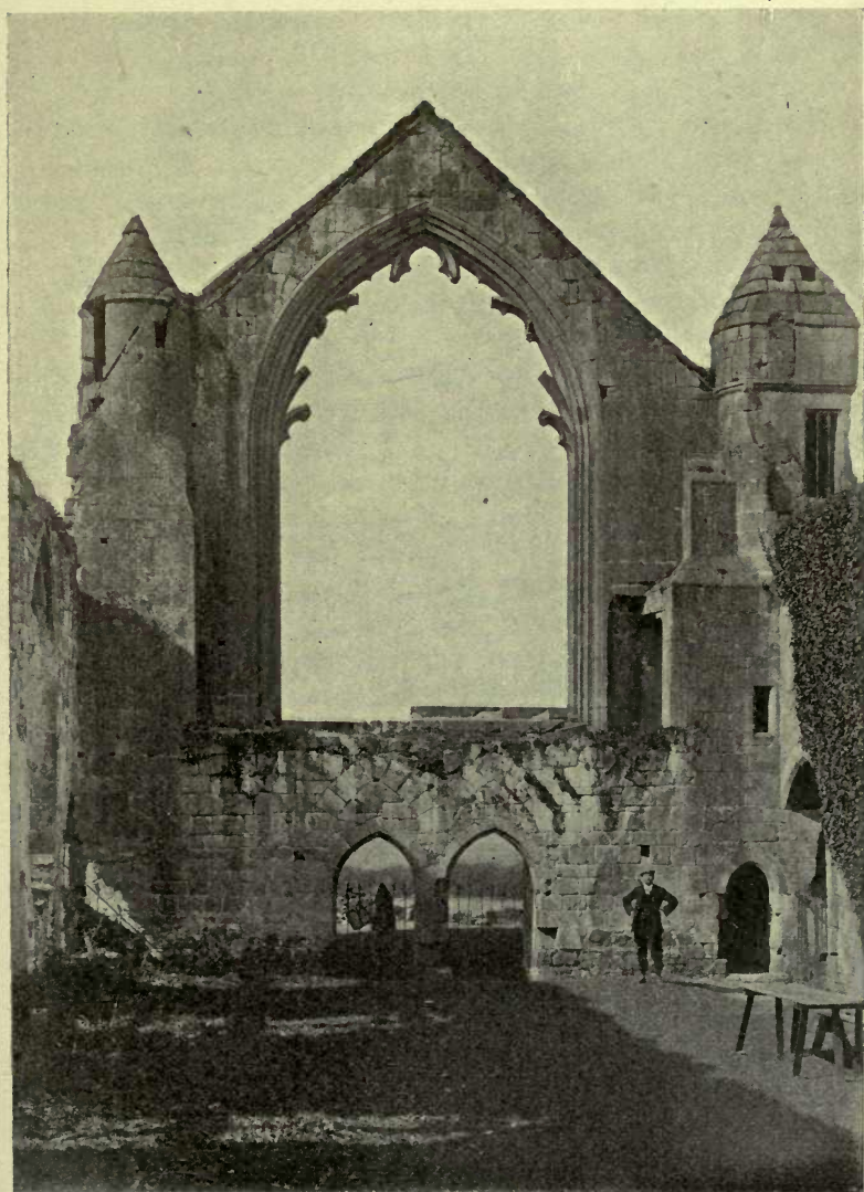
INTERIOR OF WEST END OF INFIRMARY HALL.
